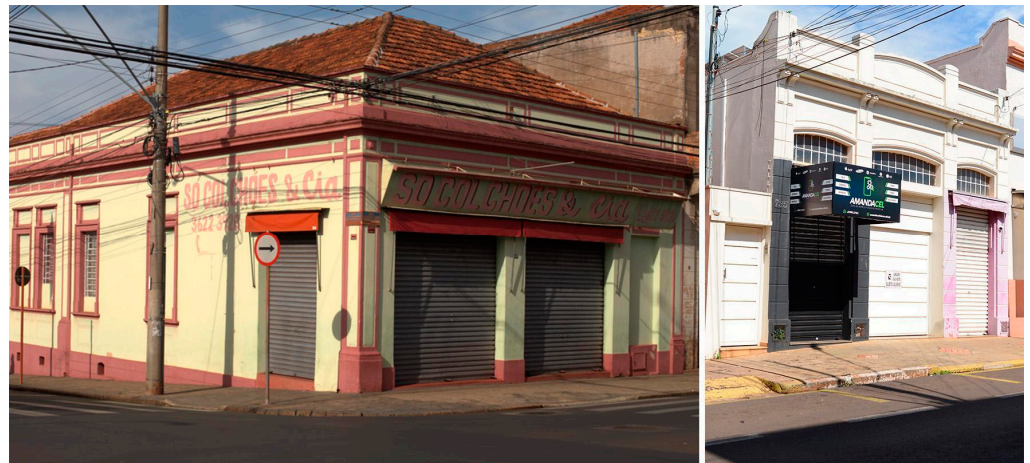
Figure 10. Examples of buildings currently characterized by significant transformations and functional adaptations. The image highlights the introduction of large ground-floor commercial openings, signage, and surface alterations, which modify the original solid–void relationships and partially obscure the compositional and decorative features of Brazilian eclecticism. Left: building in Rua Sebastião Ribeiro 576, corner building with extended shuttered openings and applied signage. Right: building at Rua Lourenço Prado 737, façade with altered ground-floor access and superimposed contemporary elements. Photo source: authors.
