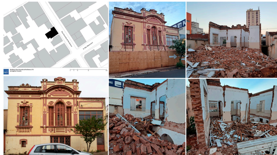
Figure 2. Images of the documented collapsed historic civic building located at Rua Visconde do Rio Branco, 273, São Carlos. Image processing by the authors.
