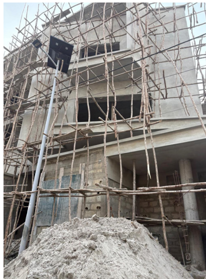
Fig. 3. Scaffoldings, Cotonou. ©Choplin, 2026
