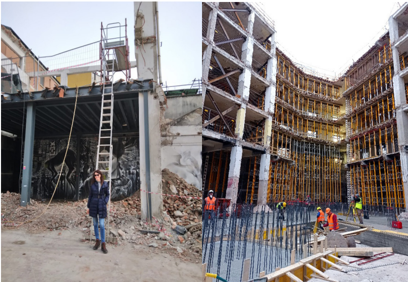
Fig. 1 Participant observation at construction and demolition sites. Source: photos by the author.
